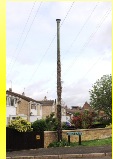
Victorian Stink pipe Bury Lane
